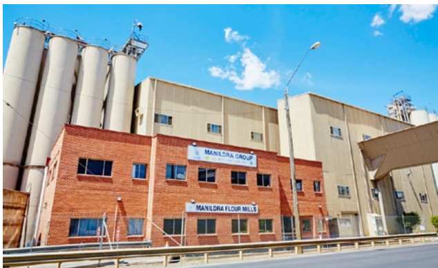
This flour mill is in the town of Manildra in the Australian state of New South Wales.
