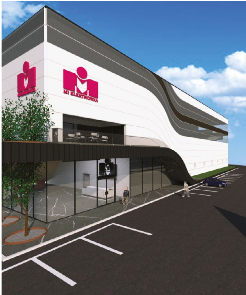
MI Elektronika is building a new plant where they plan to move the current production. Their aim is to have 250 employees by 2030.
