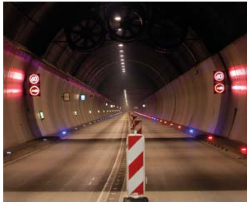
Tensor was involved in equipping Karavanke tunnel
